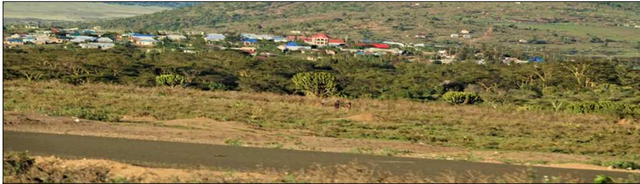
The new Musoma (Lake Victoria) to Arusha highway with the town of Wasso in the back ground, Oct. 2019
