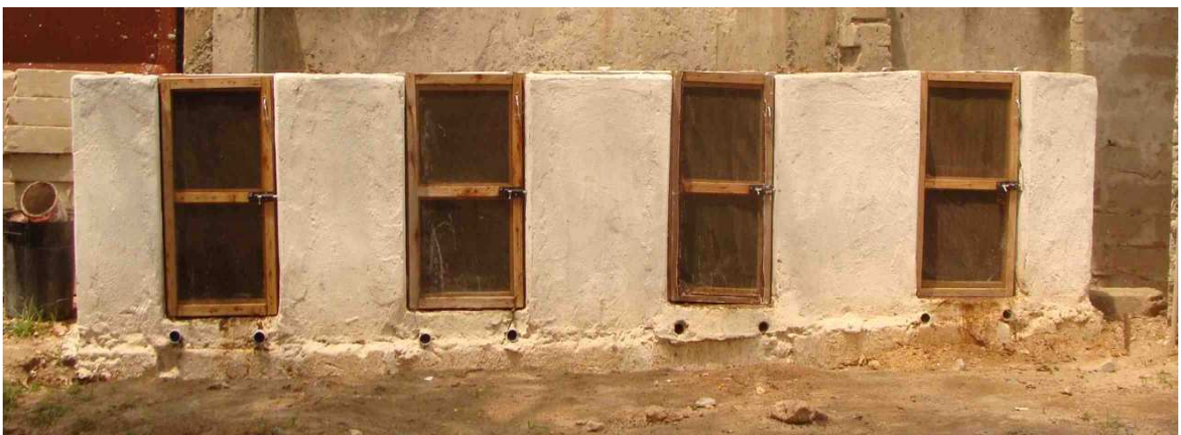
Composting chambers constructed by students and staff at Mikocheni A Vocational School.
